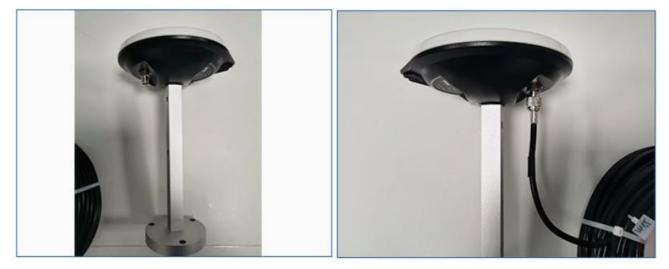
① The feeder joints need to be wound with waterproof self-adhesive tape, starting with the lower part of the joint connection and filling the low-lying part with the tape.
